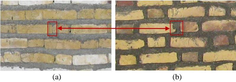
**Figure 4.** Construction detail of head joints (a) Unfilled head joint (b) Filled head joint
