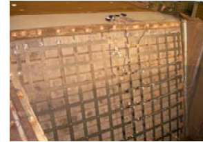
Simply reinforced masonry
