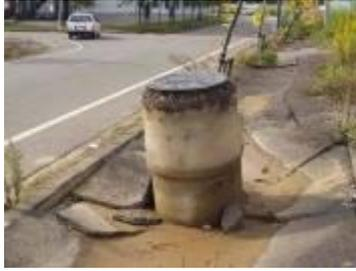
**Figure 1.** Uplifted sewage manhole during the 2004 Niigataken-chuetsu earthquake
