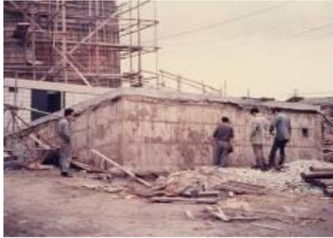
**Figure 2.** Uplifted sewage tank during 1964 Niigata earthquake
