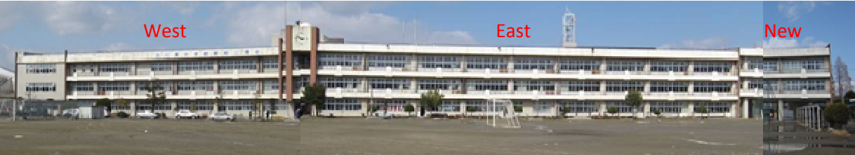
Photo 1. South view of damaged school buildings
