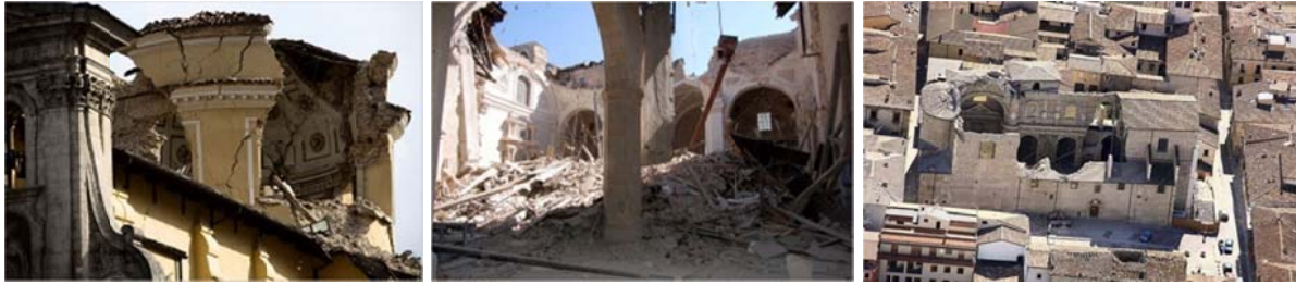
Figure 1. Damage to the architectural heritage in L'Aquila earthquake: (a) Church of Santa Maria del Suffragio; (b) Church of Santa Maria di Collemaggio; (c) Church of Santa Maria Paganica
