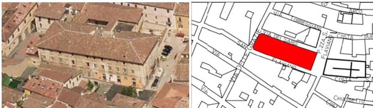
Figure 2. Aerial view of the façade on S. Flaviano St. and general plan of the building location
