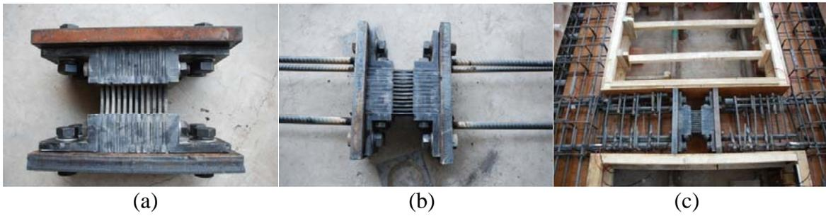
**Figure 3.2** Installation: (a) Sample damper; (b) Anchor rebars; (c) Installation in the framework
