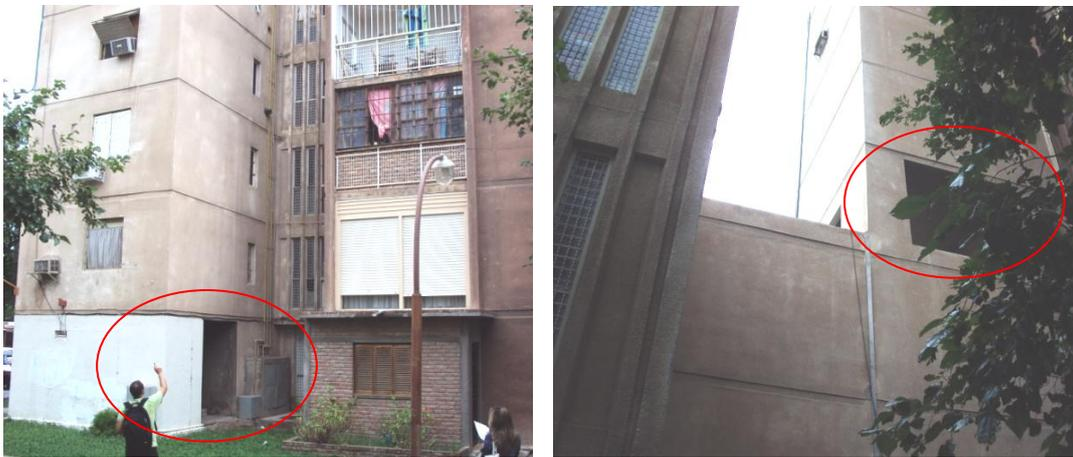
**Figure 4.** Discontinuity walls in the first and fourth floor.
