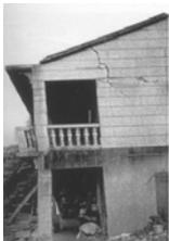
**Figure 7.** Building leans forward due to foundation settlement (Chang, J. S. et al., 2001)
