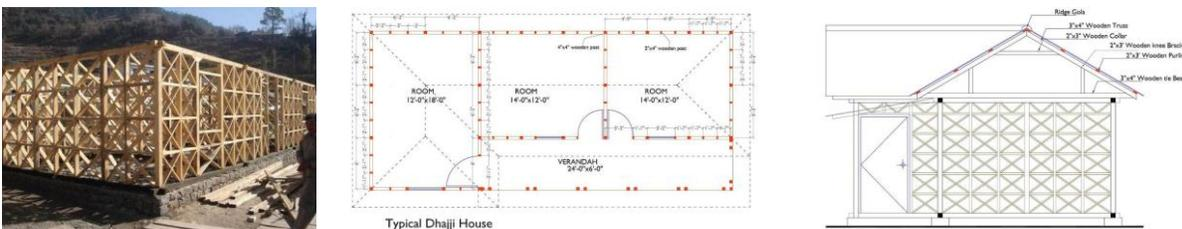
Figure 2. "Engineered" Dhajji building frame under construction in Pakistan.
