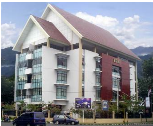
(a) Before earthquake damage
