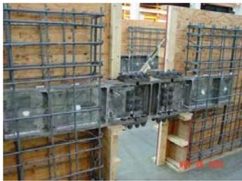
**Figure 1.3.** As-built details of replaceable coupling beams( Fortney, 2005)
