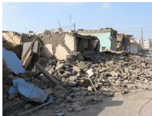
Figure 1. Destruction of adobe houses Pisco, Peru. 5/08/2007 (Photo: Eric Hulburd)
