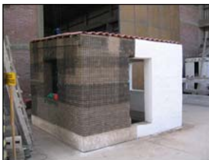
Figure 4. Model reinforced with geogrid, half plastered
