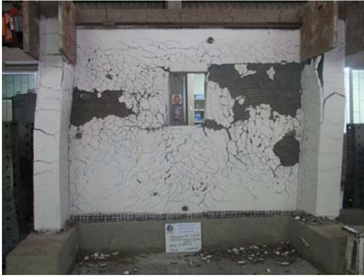
Figure 7. Cyclic shear test on reinforced adobe wall.
