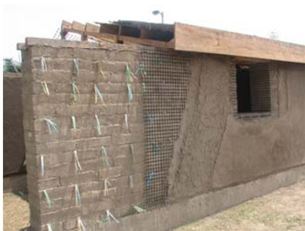
Figure 3. Construction process of geogrid reinforcement
