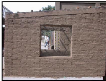
Figure 6. Plastered side after testing.
