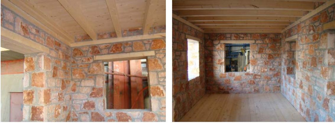
**Figure 2.** Photos of the wooden slabs and the lintels
