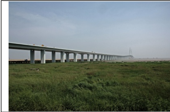
Figure 3. Hangzhou Bay Bridge, Most L is Low-Level Viaduct, Total L=35.673 km, China, Opened in 2008.
