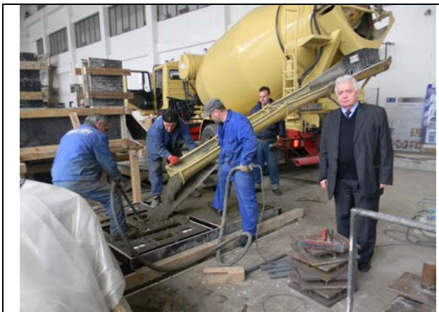
Figure 9. Construction large-scale experimental bridge model in IZIIS, Skopje dynamic testing laboratory
