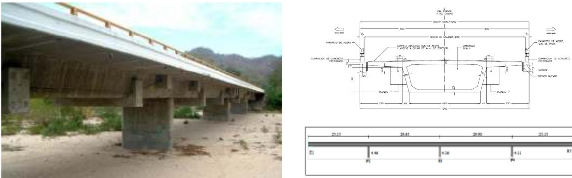
**Figure 1.** Photograph and general dimensions of Motín de Oro Bridge
