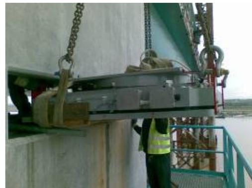
**Figure 3.** Monitored fixed spherical bearing. Calibration and Installation phases.
