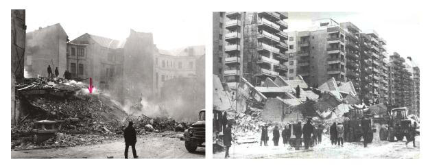
Figure 2. Full collapse and extreme loss of volume in 1977 in case of pre-1940 RC structure, Al. Sahia No. 1-3, (left) and collapse of pre-1977 OD 16 Block shear-wall section (right).
