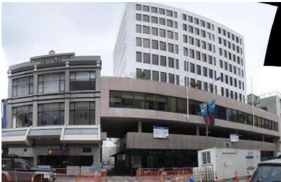
Figure 11. Minor damage to adjacent building with different height., Christchurch
