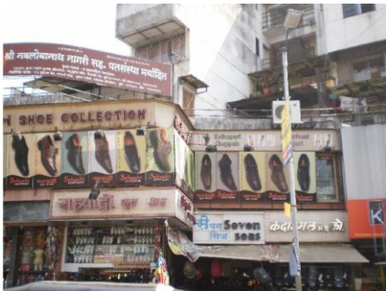
Figure 12. Adjacent building with different heights Pune.
