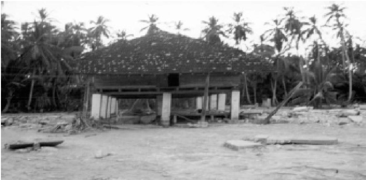
**Figure 3.3** A rectangular timber hut supported on plain concrete columns.
