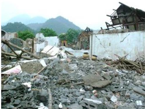
Figure 5: Damaged wooden/brick houses, 2008 (China)
