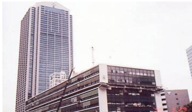
**Figure 8:** Damage of Kobe City Hall, 1995 (Japan)
