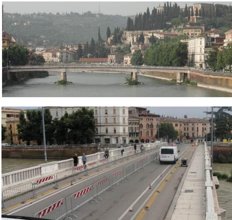
Figure 1. – The analysed bridge (photo 2011).
