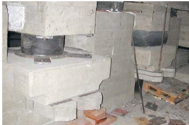
Figure. 1 Installed new and old bearing
