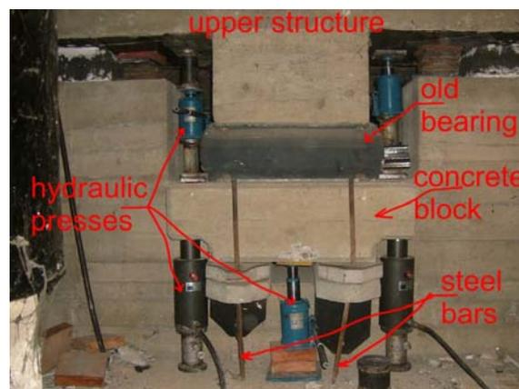
Figure 5. Placement of the hydraulic presses
