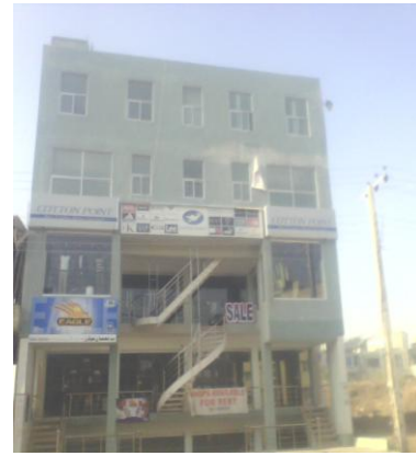
Figure 2. Real Picture of Building in Pakistan for which Seismic evaluation is performed
