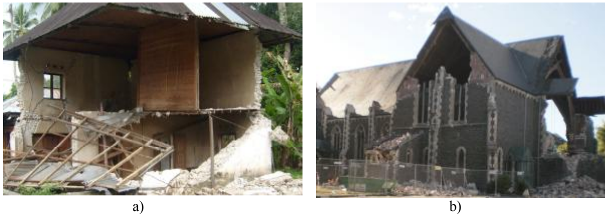
Figure 4.3. Out-of-plane collapse of stone masonry walls: a) the 2009 Padang, Indonesia, earthquake (Bothara et al. 2010), and b) collapse of gable walls in the 2011 Christchurch, New Zealand, earthquake (photo: J. Bothara)
