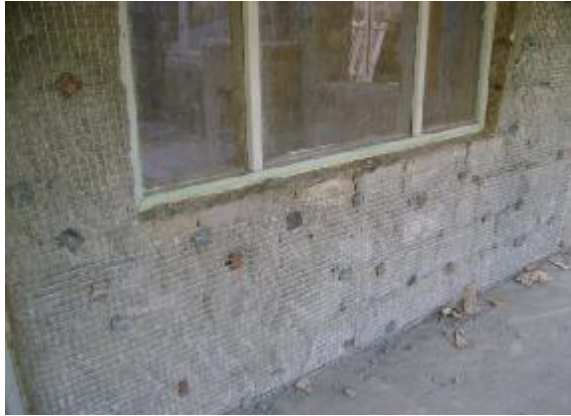
Figure 6.2. Jacketing of stone masonry walls in Pakistan after the 2005 Kashmir earthquake: a) a wall surface showing reinforcement and anchors in place before the plaster application (photo: Q. Ali), and b) a detail of steel mesh reinforcement and through-wall anchors (photo: T. Schacher).
