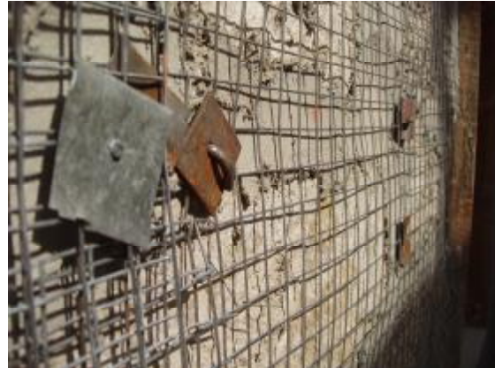
Figure 6.2. Jacketing of stone masonry walls in Pakistan after the 2005 Kashmir earthquake: a) a wall surface showing reinforcement and anchors in place before the plaster application (photo: Q. Ali), and b) a detail of steel mesh reinforcement and through-wall anchors (photo: T. Schacher).
