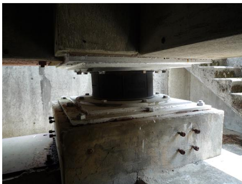
Figure 2. Detail of the rubber isolator
