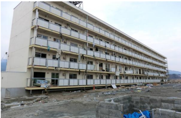
Figure 1.1. Survived a Five-story Concrete Building at Rikuzentakada, Iwate Prefecture in Japan(2011)
