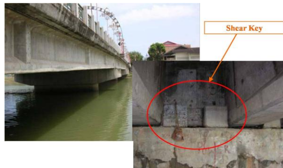
Figure 1.4. Survived the Concrete Bridge at Banda Aceh in Indonesia (2004)
