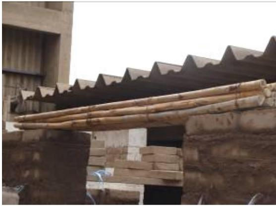
Flexible cane roof lintel and cover fiber-cement sheets
