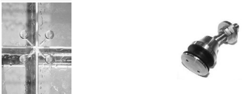
**Figure 2.1.** Point fixed glazed façade system: Left) example of a point fixed façade; Right) example of a bolt used to perform the panel's support (Martins 2011)
