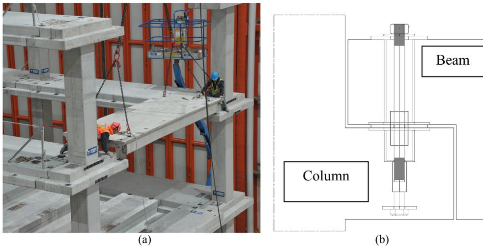
**Figure 3.** (a) Seating of a secondary beam on the column capital. (b) Detail of a pinned beam-column joint connection and a dowel with increased diameter at the critical section.
