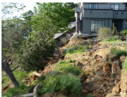
Figure 1. Fill slope failure. (The 2011 off the Pacific coast of Tohoku Earthquake) Left panel:valley axis direction. Right panel:valley cross-sectional direction.
