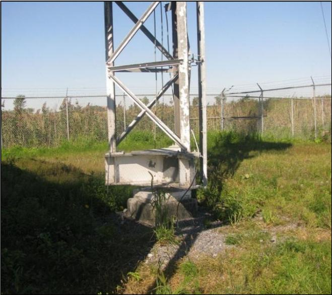
b) Mast pinned-base connection
