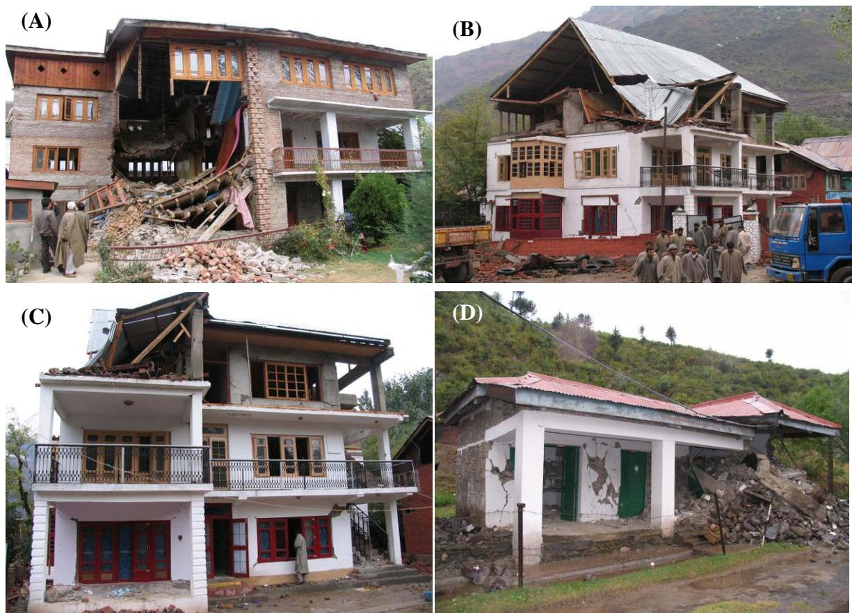
**Figure 1.** Damage observed in hybrid buildings in the Kashmir earthquake, 2005 (photo courtesy: CVR Murty)
