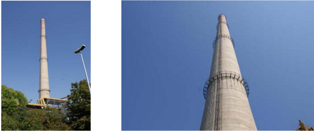
Figure 1. Power plant “Negotino chimney
