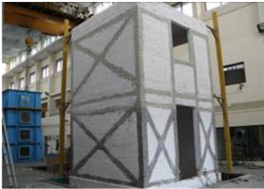
Figure 4.1. Clay brick building with stripe application (east – north side)
