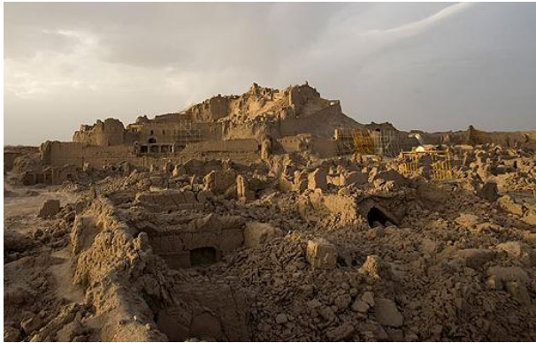
Figure 1.3. The citadel of Bam after the earthquake of 2003 (6.2 degrees on the Richter scale)
