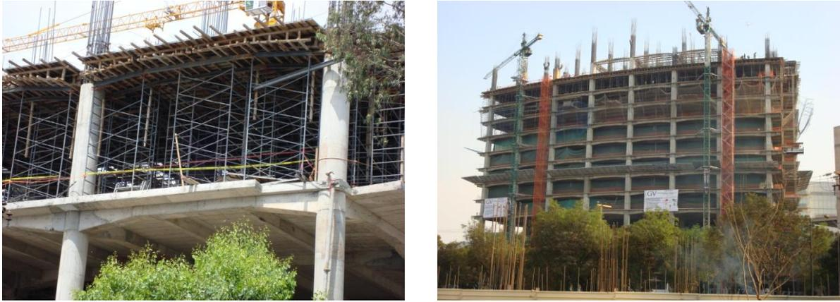
**Figure 3.1.** Reinforced concrete buildings with haunched beams under construction in Mexico City
