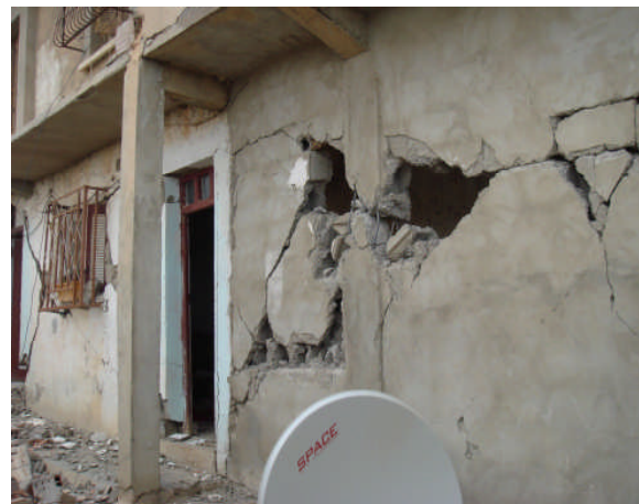
Figure 4.6. Masonry-structure interaction and bad quality of design and execution
