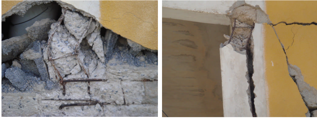
Figure 4.9. Inadequate proportioning and detailing of structural elements
