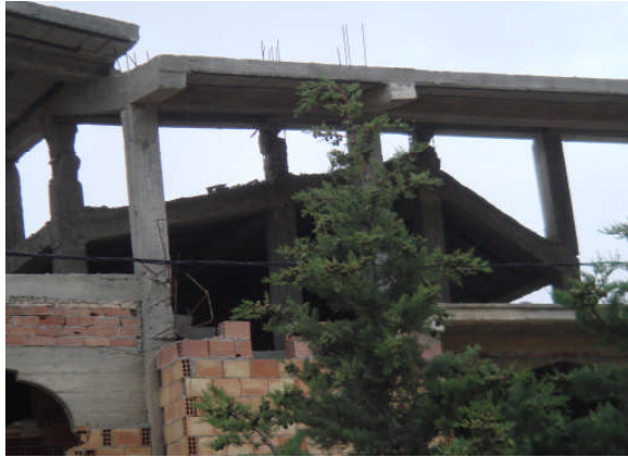
Figure 4.3. Short columns
