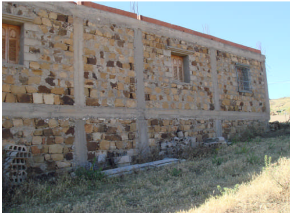
Figure 4.2. Confined bearing masonry structures (one school and three houses) that behave very well.
