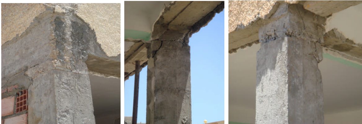
Figure 4.8. Poor quality of execution and inadequate concrete recasting
