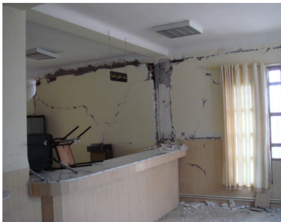
Figure 4.6. Masonry-structure interaction and bad quality of design and execution
