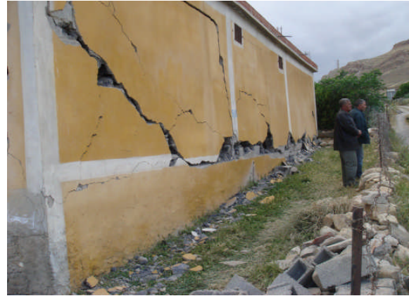
Figure 4.4. Vertical dissymmetry and poor quality of execution
