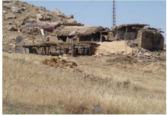
Figure 4.1. Collapse of non confined bearing masonry structures
