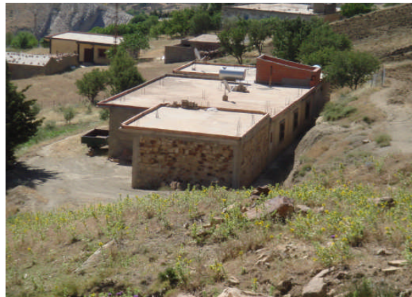
Figure 4.2. Confined bearing masonry structures (one school and three houses) that behave very well.
