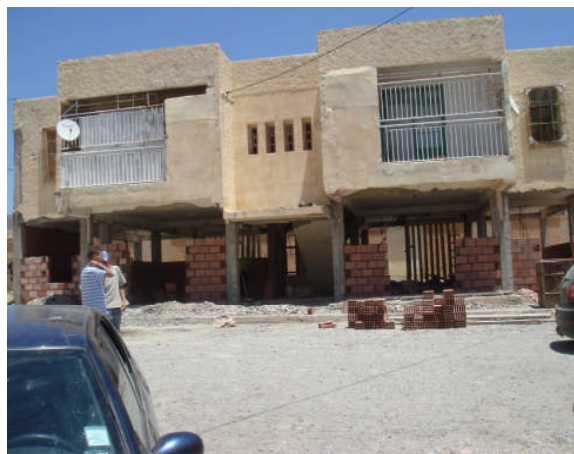
Figure 4.5. Soft story (Classroom at the 1 st story under rigid apartment 2 nd story)
