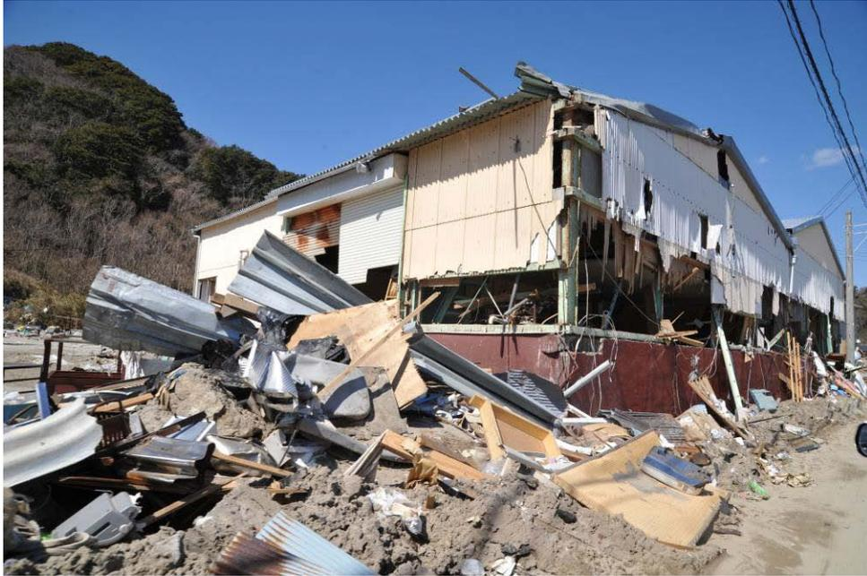
**Figure 1.** Total destruction, deformation and movement of steel structures in Onagawa town, Japan 2011 (Vulnerability Class C, Grade 5) (Intensity: XII).
