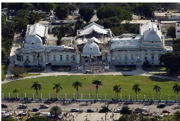
Figure 1. Damaged Presidential Palace in Port-au-Prince (UNDP Global 2010).
