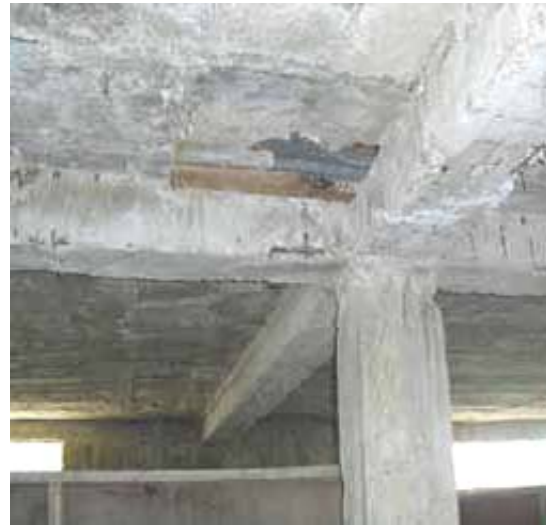
embedded formwork and exposed reinforcing
