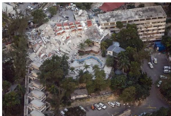
Figure 2. Collapsed UN building in Port-au-Prince (UNDP Global 2010).
