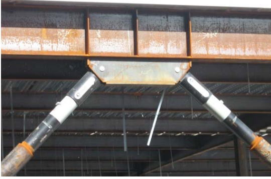
Figure 1. Steel moment frame with dampers
