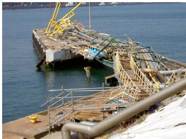
Figure 4. Berth collapsed by a ship strike
