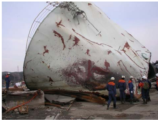
Figure 3. Oil storage tank drifted and collapsed by the tsunami
