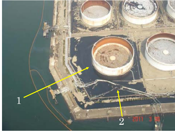
Figure 2. Heavy oil spilled in the dike
