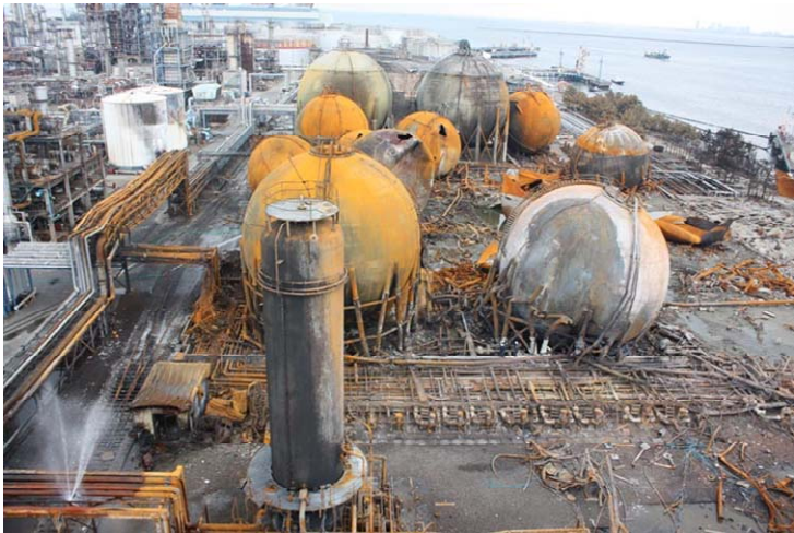
Figure 14. Burned and exploded LPG tanks at Ichihara
