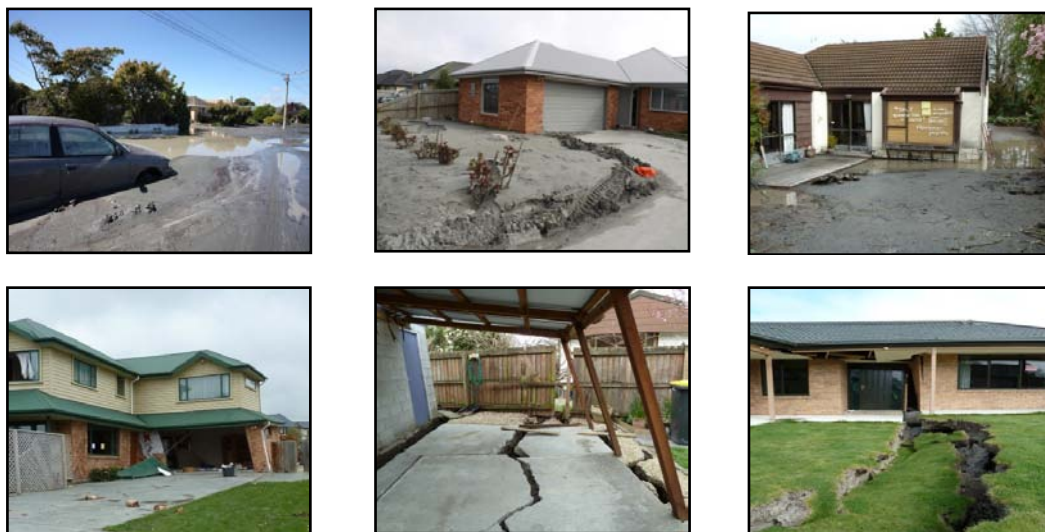
Figure 2. Examples of land and building damage
