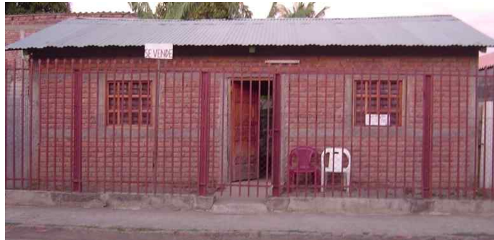
Figure 3.1. Non-engineered concrete frames with infill bricks in Rivas, Nicaragua
