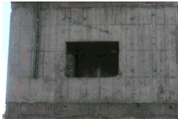
**Figure 1:** Concrete shear wall with opening (Iran; Semnan 2011)
