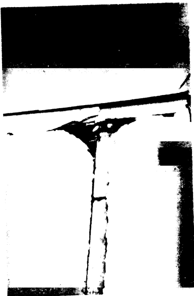
Fig. 3 Damage to nonstructural walls as well as to structural elements. (Note the width of the "equivalent" diagonal)
