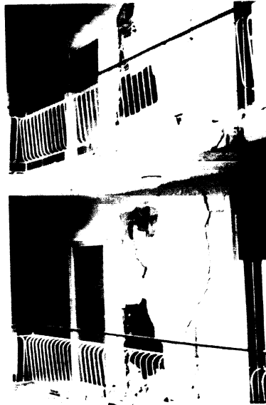
Fig. 2 Damage to nonstructural facade walls
