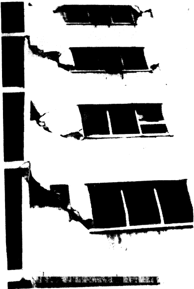
Fig. 2 Damage to nonstructural facade walls
