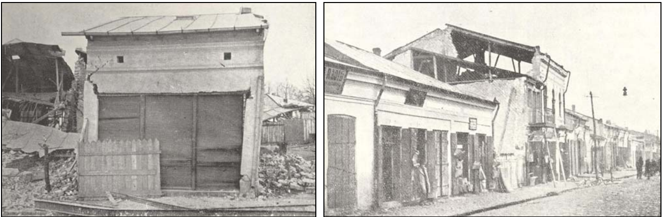
Figure 2. Damage of dwellings in Panciu and Adjud towns, 1940 (Niculescu, 1941).
