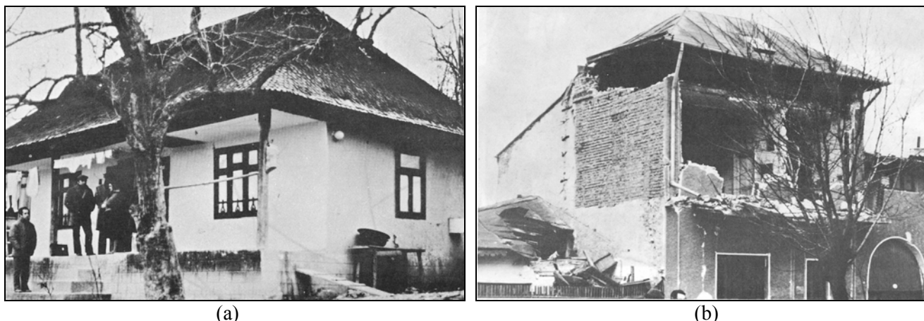
Figure 4 (a). Typical one story adobe/wood wall dwelling in Vranceaia. (b). Typical old two-story unreinforced masonry wall dwelling, Bucharest, 1977 (Rojahn, 1977).
