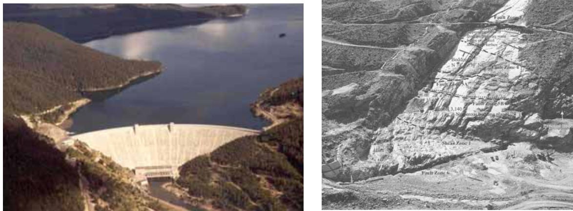
Figure 1. General View of Hungry Horse Dam and continuous bedding plane partings - left abutment
