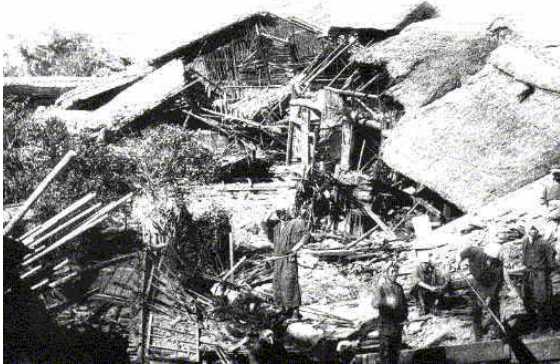
Photo 1: Damage of timber houses and new brick factory (the 1891 Nohbi Earthquake)
