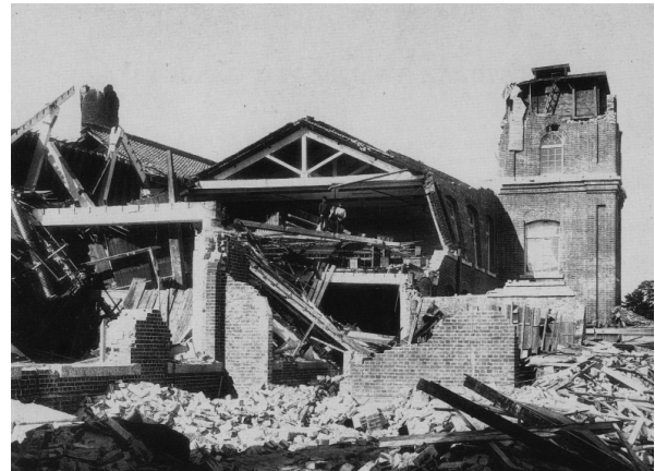
Photo 1: Damage of timber houses and new brick factory (the 1891 Nohbi Earthquake)
