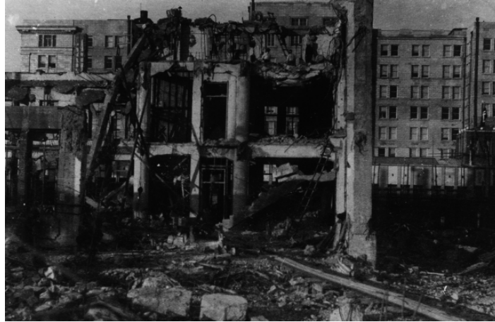
Photo 2: The Naigai Building near completion collapsed
