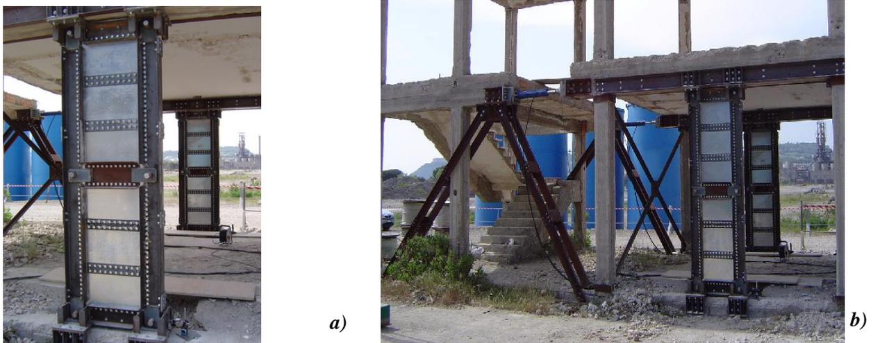
Figure 5 Steel (a) and aluminium (b) shear walls inserted into the RC frame structure
