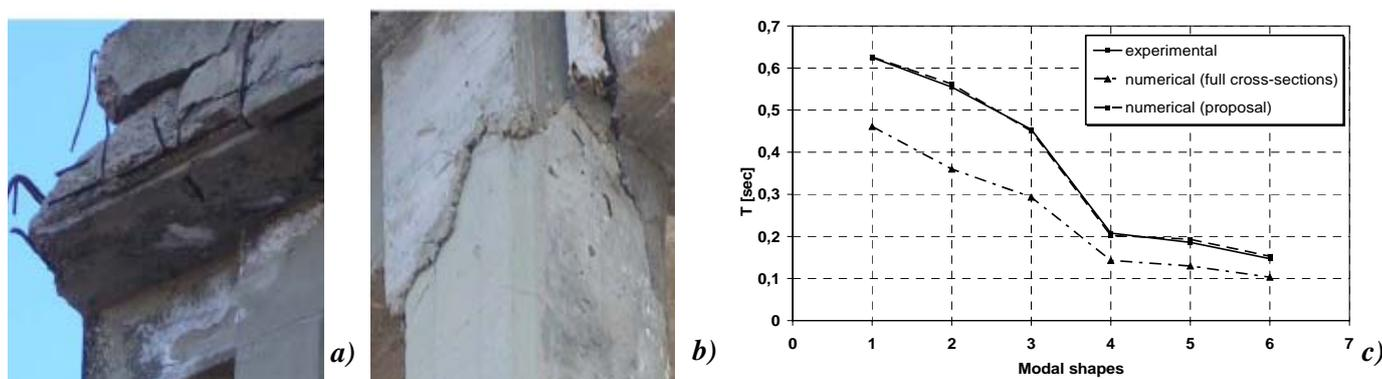
Figure 4 Beam (a) and column (b) degradation and experimental - numerical comparison in terms of vibration periods (c)
