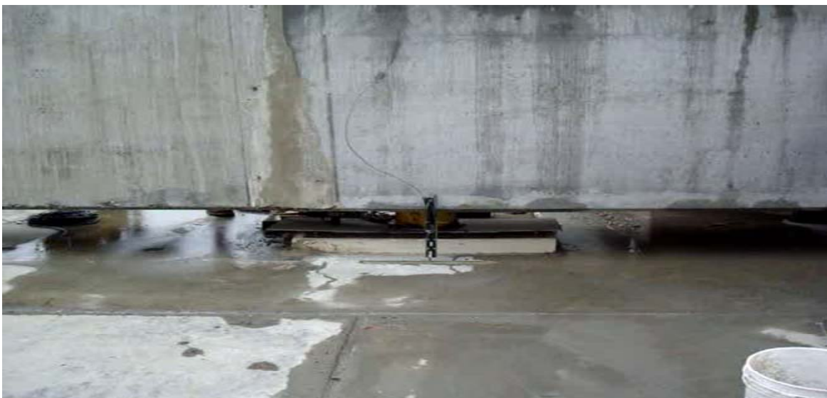
Figure 11 Photograph of one external beam showing one supporting Seismic Filter.
